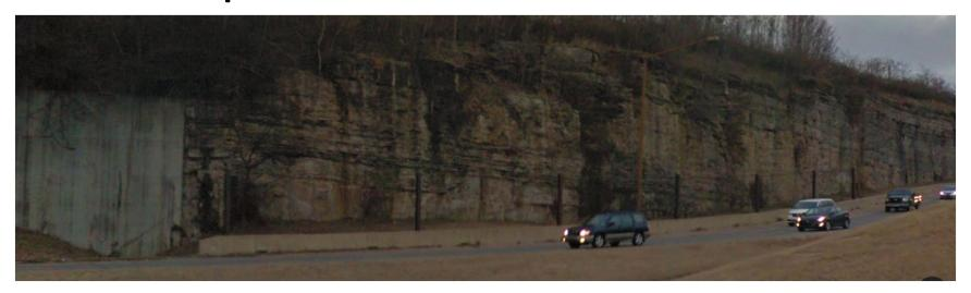
Minor Damage to Rock Fence Panels, Panels bulge inward and outward, Catchment Relatively clean.
